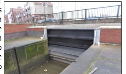
Planks in use, December 2016
