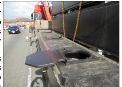
Valve flaps in one of the stop planks
