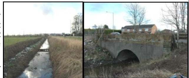
Traces of the canal can still be seen alongside the A5104 in Saltney with a bridge under the road close to Morrisons.
