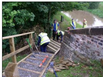
Installing Stepped Access at Calveley
